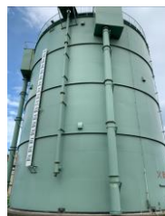
Biogas holder (gas adsorption, refining)
