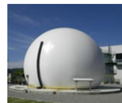
Biogas holder (receiving tank)
